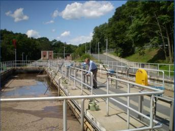
Nitrification – Ammonia (NH<sub>4</sub>) removal – eliminate influent and RAS flow into tank when air is ON ... Less BOD to compete with nitrification More HRT to allow for effective nitrification
