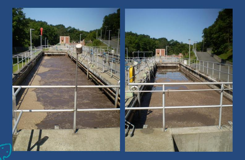
Using ORP as the process controller, every  $1-1\frac{1}{2}$  hours, valves open and close to switch conditions in the aeration tanks, much like a Sequencing Batch Reactor
