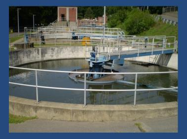
Open and Close inlet and RAS valves to ... Optimize treatment time in air ON and air OFF zones Reduce solids loading on secondary clarifiers
